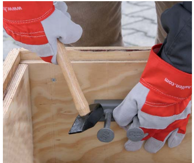
Nail the HALFEN cast-in channel to the formwork
