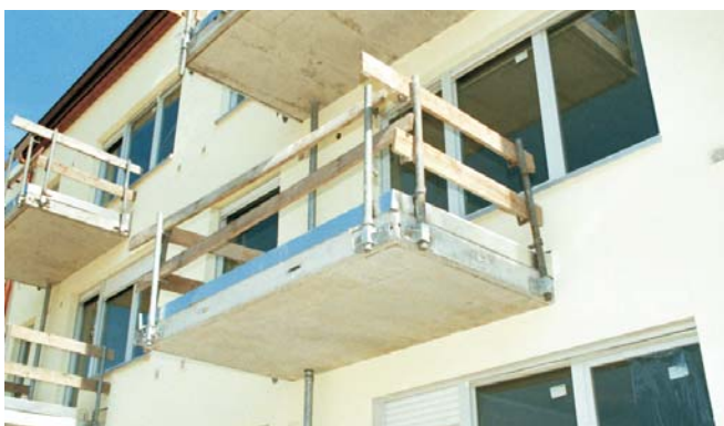
Fall protection during the construction phase
